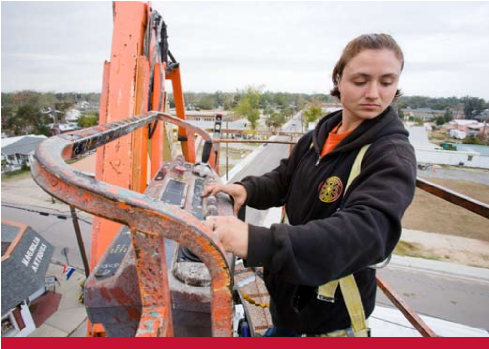
Sabrina Graley, a graduate of the Women in Construction training program, works on her first job in Bay St. Louis, Mississippi. DECEMBER 2008
